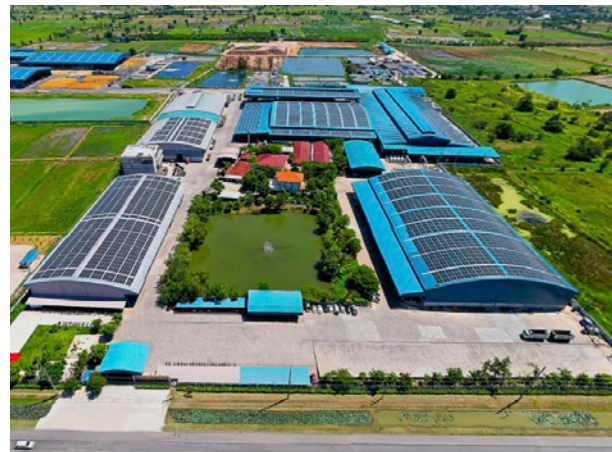
Electricity Production from Solar Energy Installed on the Roof Project
