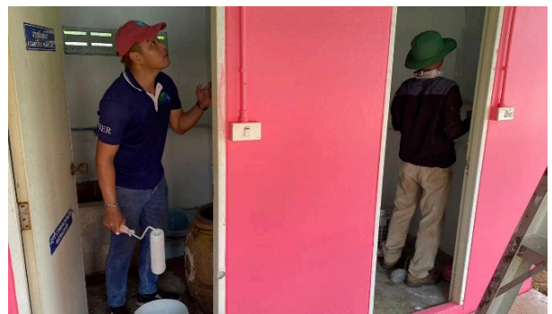
Our Employees Repainting and Repairing Ban Chai Phattana Monastery
