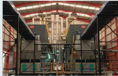
Project to replace the boiler system with a high-efficiency model
