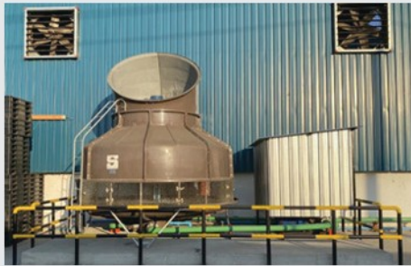
Project to replace the chiller cooling system with a cooling tower
